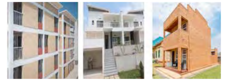
Batsinda II cement soil blocks 3-storey, 176m 2
