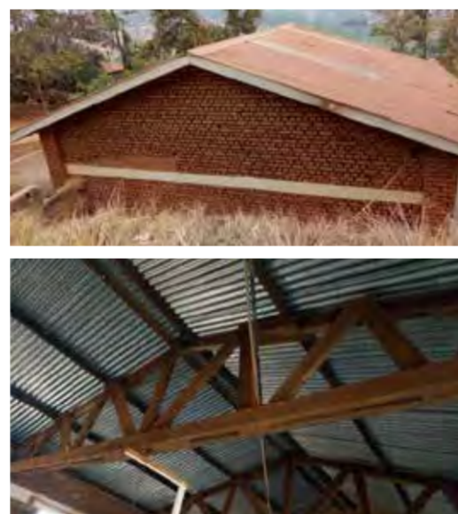
Figure 2: Office building of Biryogo Primary School from outside (left) and inside (right)
